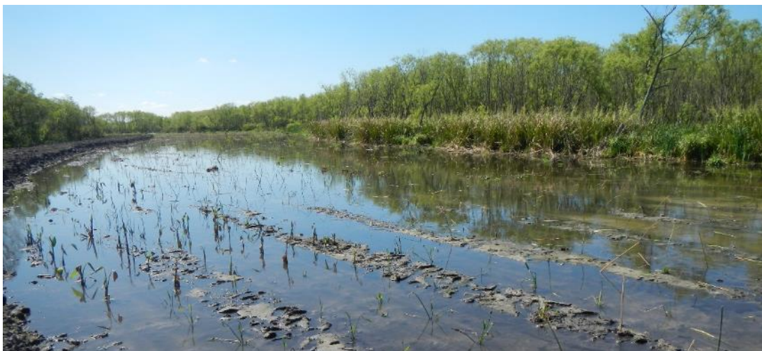
Figure 7. Sweetwater Branch/Paynes Prairie Sheetflow Restoration Project Canal Backfill
