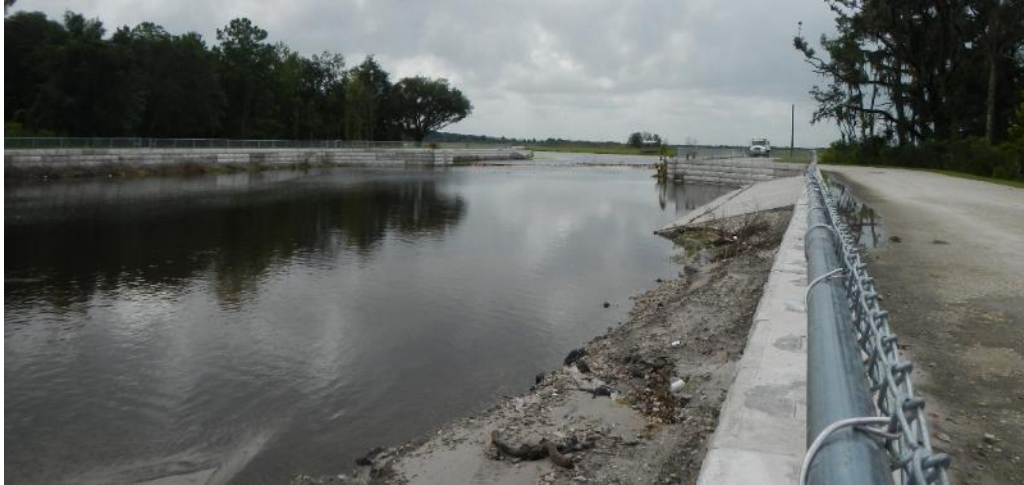
Figure 2. Sweetwater Branch/Paynes Prairie Sheetflow Restoration Project Sediment Basin
