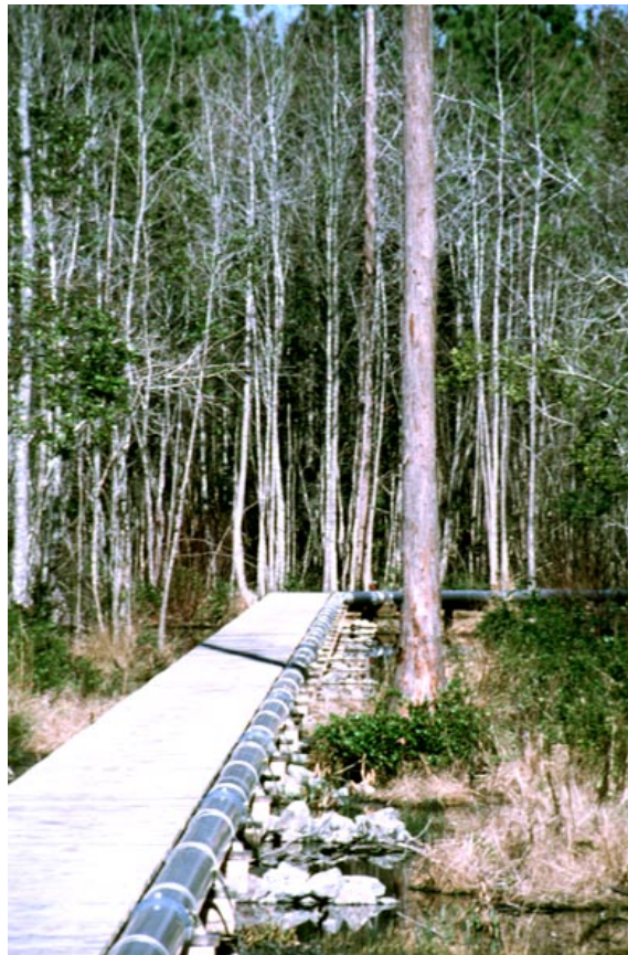
Gated pipes on raised boardwalks allow access to over 600 acres of treatment area in the Vereen Natural Treatment Wetland in South Carolina.
