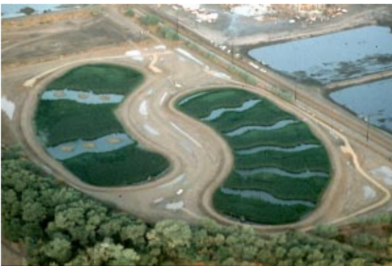
The Hayfield Site demonstration Wetland at Tres Rios west of Phoenix, Arizona, includes two cells with variable numbers of deep water zones to test their effect on hydraulic efficiency and wildlife habitat.
